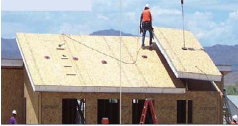
**Figure 18: Insulfoam's Structurally Insulated Panel**
