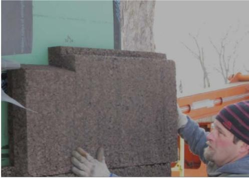
**Figure 14: ThermaCork Insulation Plus Siding**
