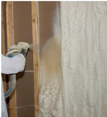
**Figure 9: Johns Manville Spray Foam Wall Insulation**
